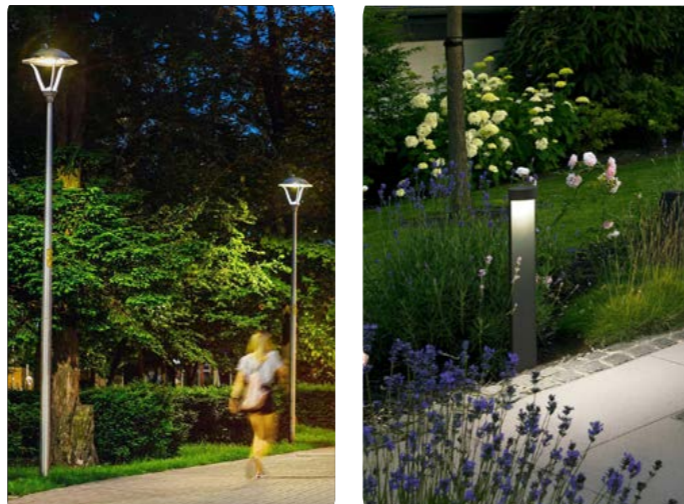
New lighting providing safe routes and low glare
