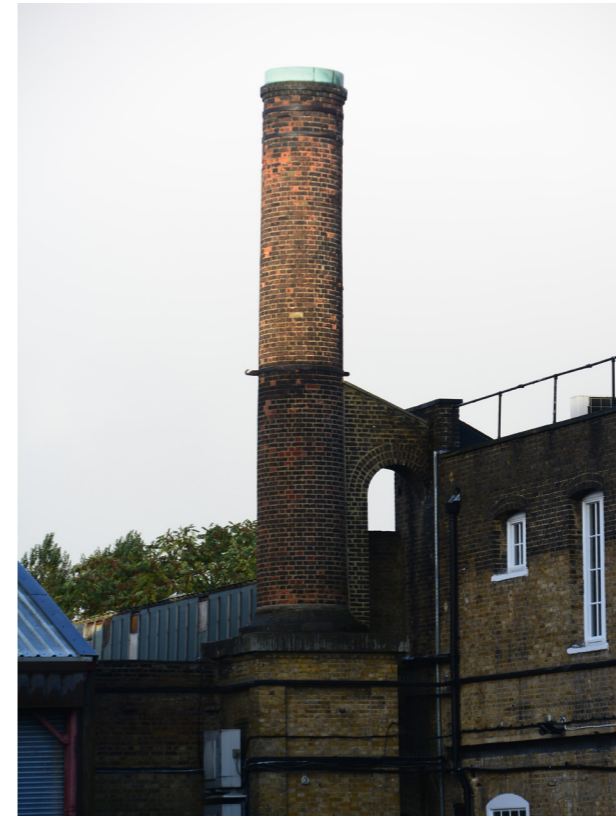
Heritage structures such as the chimney of the Cooperage should be retained.
