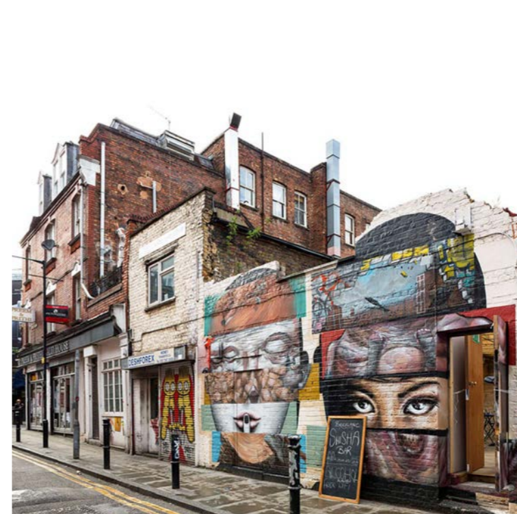
Existing Site Condition
