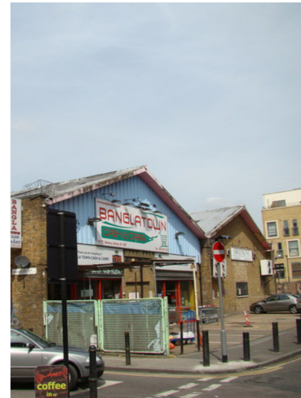
Existing condition of Banglatown Cash and Carry
