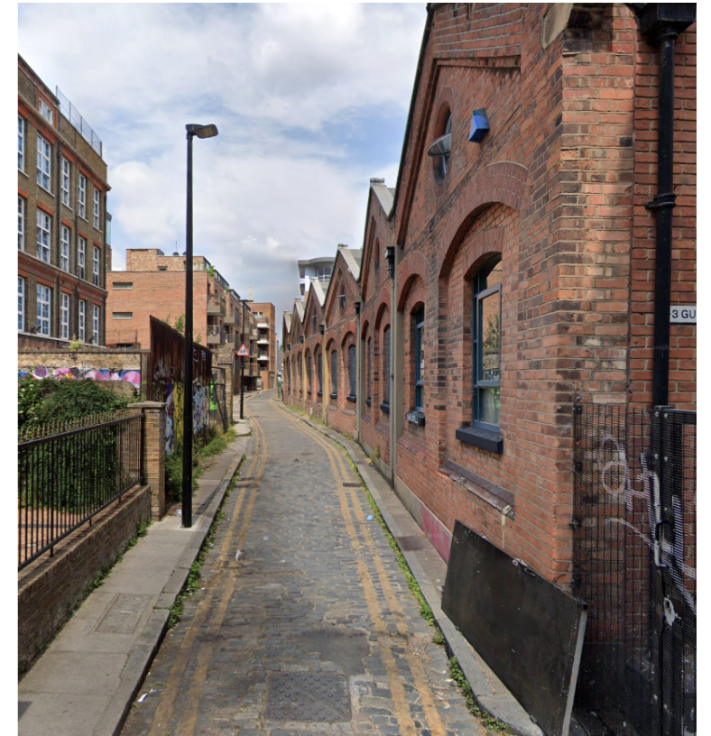
Looking North down Gunthorpe Street at the rear of the site
