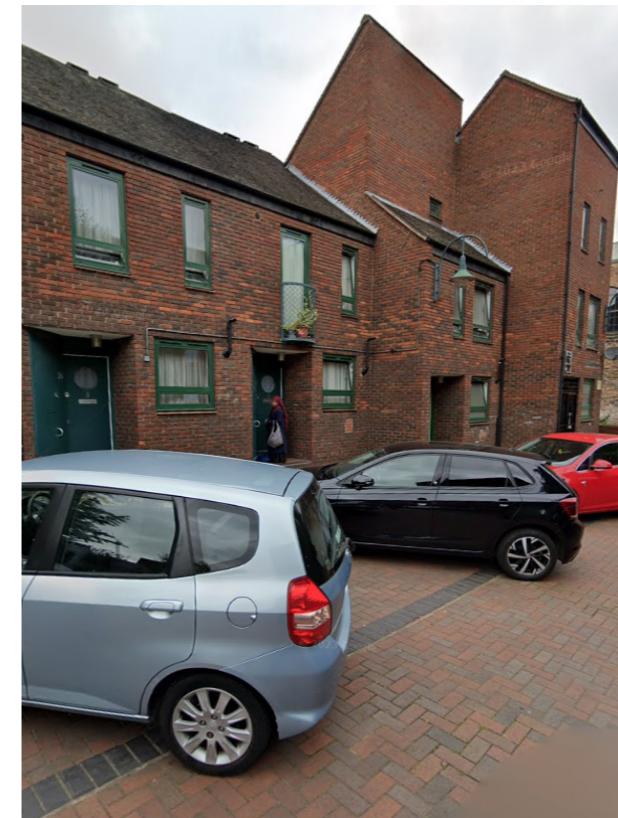
Existing condition of housing on Flower and Dean Estate
